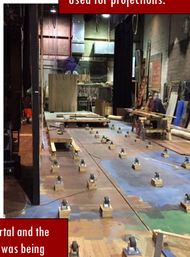
Below are behind-the-scenes pictures of the set as it was being built. The train set operates like a giant skateboard that rides on top of wheels bolted to the stage floor. As the scene shifts from one section of the train to the next, the "train" is pulled/pushed to the open section on view in the portal. The portal screen is also used for projections.
