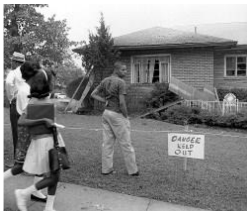
Bomb-damaged home of Arthur Shores, September 5, 1963
